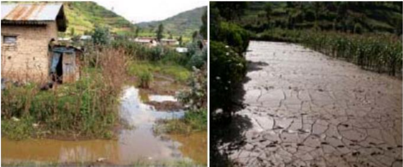
Figure 20 : A farm and a house near Gishwati forest damaged by floods
