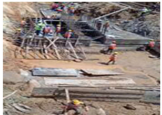
Construction works at Intake of Ntaruka A
