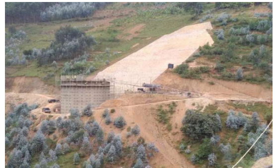
Surge Tank Construction for Rukarara
