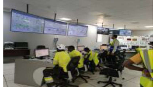
Testing and commissioning at Hakan
