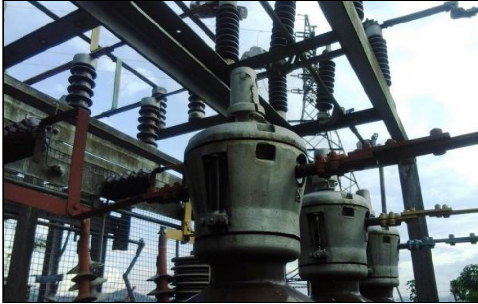
Fig. 4: Cracked CT for one of the Outgoing 30kV Feeders.
