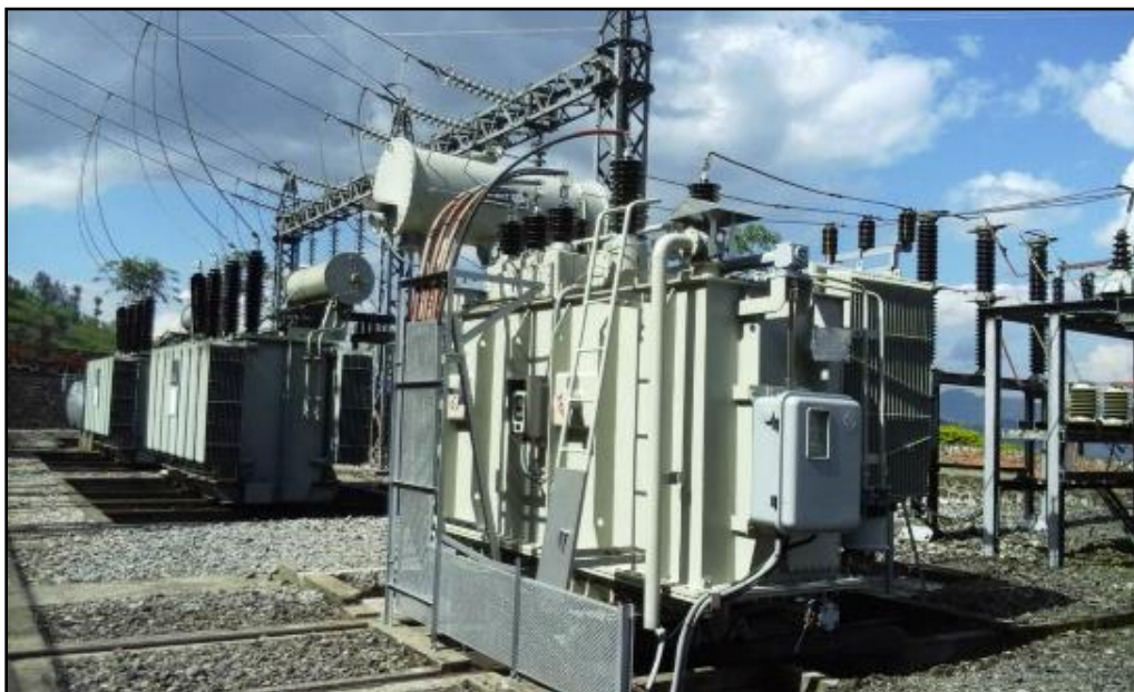
Fig. 2: Part of the Outdoor Substation/switch yard “three outdoor transformers” at Ntaruka.
