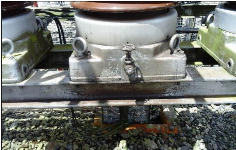
Fig. 5: Oil Seepage on a CT for one of the Outgoing 30kV Feeders.
