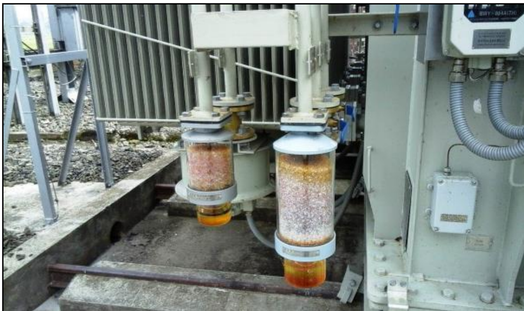
Fig. 3: Deteriorated Silica Gel.
