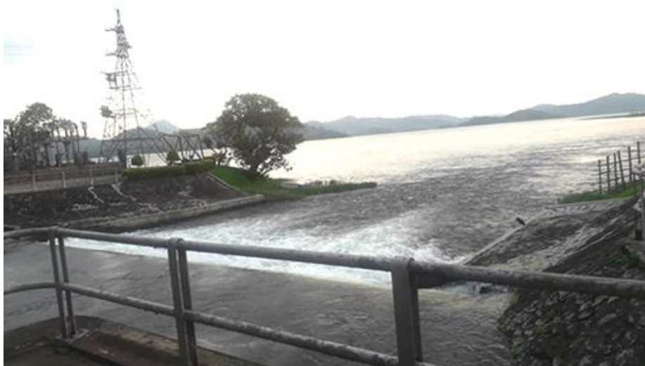
Fig. 15: Outlet of Ntaruka Hydro power plant into Ruhondo Lake
