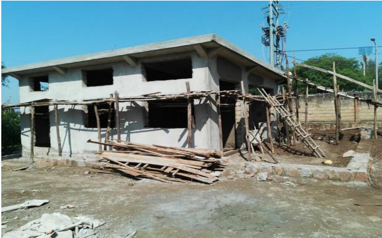
Six cabin status in January 2017
