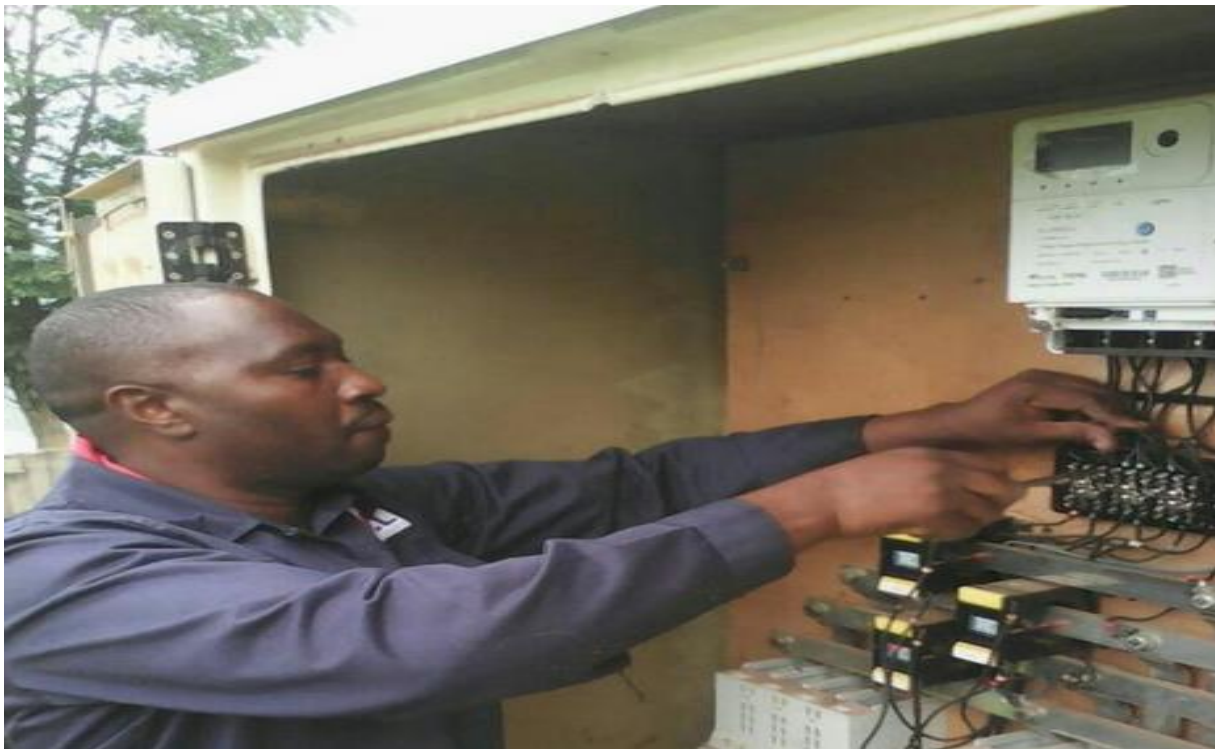
Installation of smart meters “prepaid meters’
